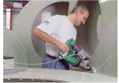
The FUSION 2 in operation during container construction.
